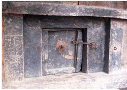
Kothars* for storage of grains and unique type of locking system in "Kolhar" Photo by, Sofia Camalin
